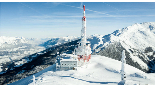
Fig.: Wind measuring station Patscherkofler
